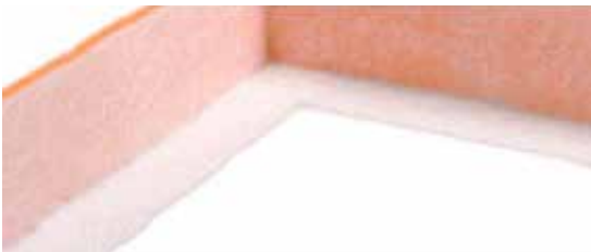
Fixing insulation strip to walls.
