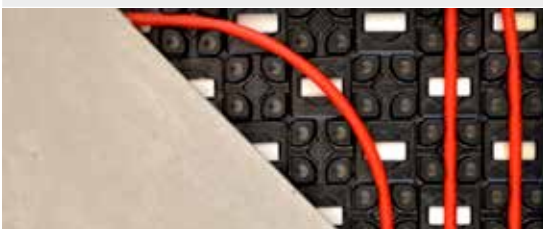
Pouring filling compound.
